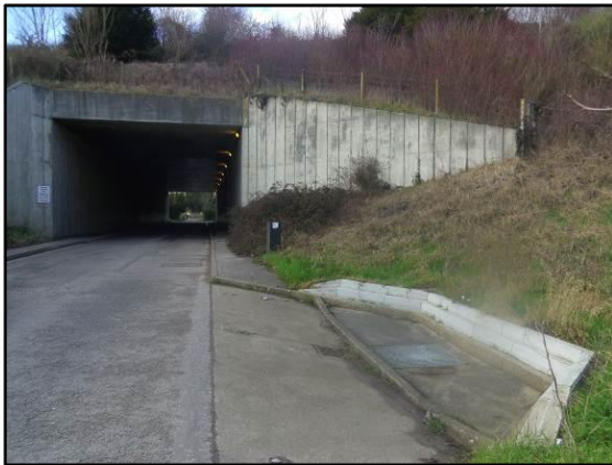
Photograph 5.34: Super Gully by A27 Underpass (looking north)
