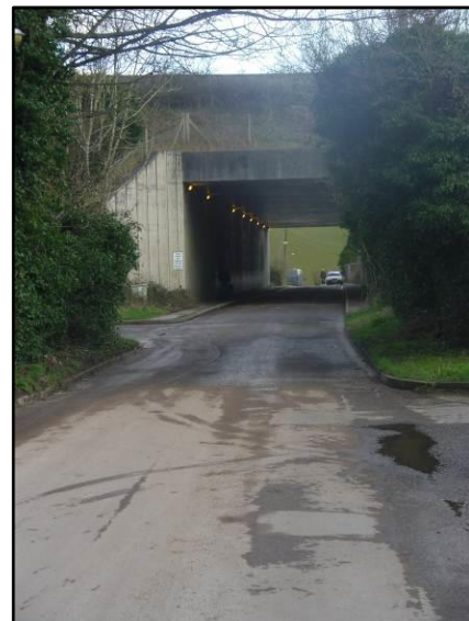
Photograph 5.33: A27 Underpass (looking south)
