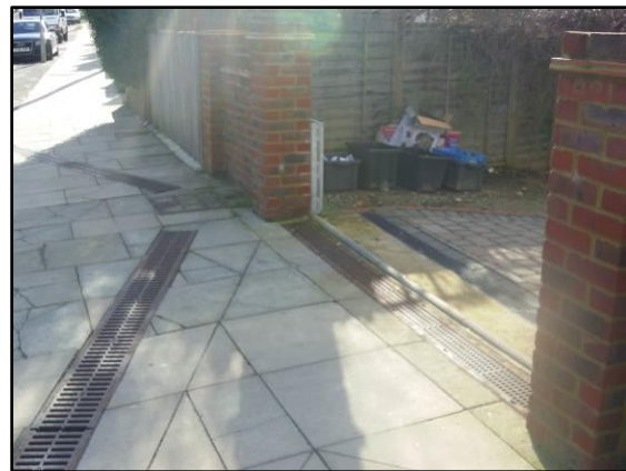
Photograph 5.30: Slot drains and flood gate
