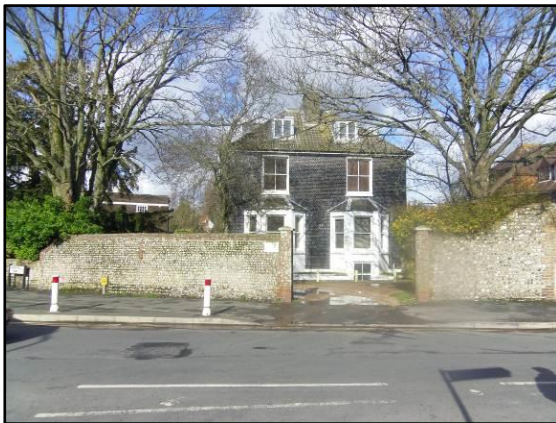
Photograph 5.26: Basement Properties at 94 Old London Road property)
