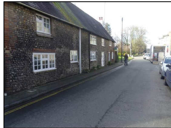
Photograph 5.27: 54-57 Old London Road (steps down into property)
