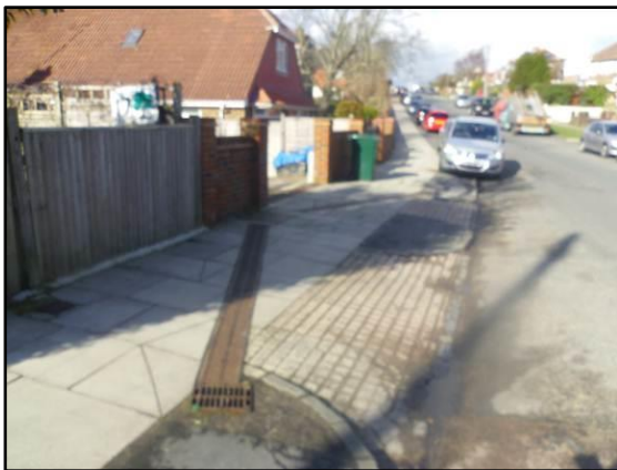
Photograph 5.29: Gullies and Slot drains outside 17a Warmdene Road
