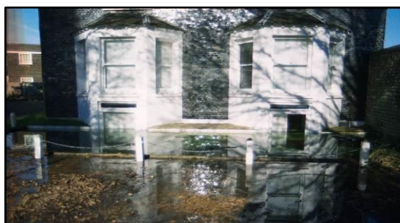
Photograph 5.21: 94 Old London Road (2000)
