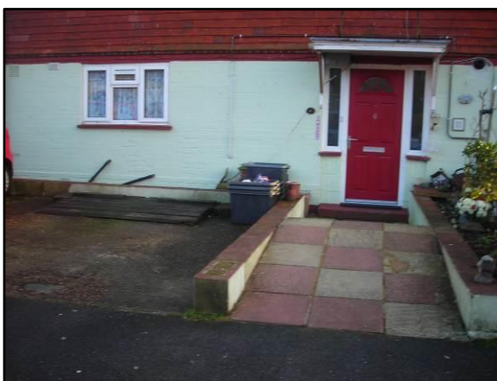
Photograph 5.12: Property Level Protection to house in Bodiam Close
