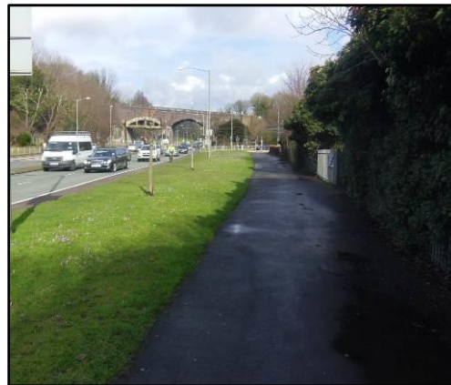
Photograph 5.7: Pavement adjacent to school
