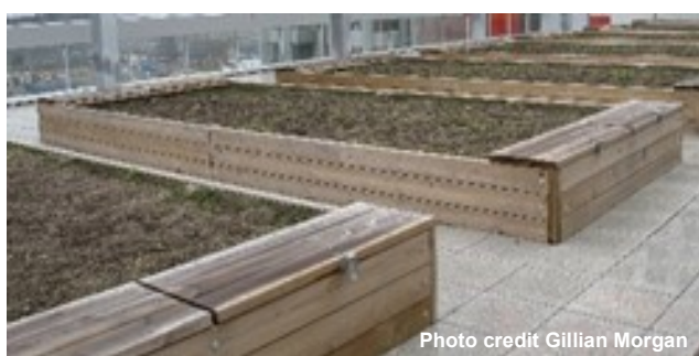
Storage areas and seats built into the ends of raised beds
