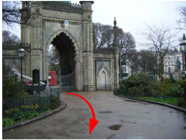
General view inside of William IV Gate.
