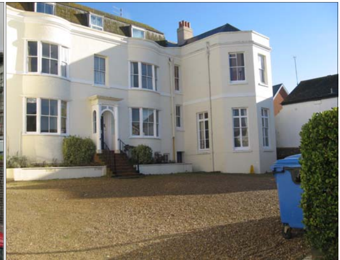
Small car parking area
