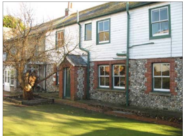
Curtilage listed terraced cottages
