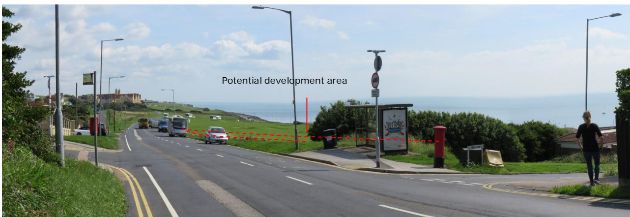
View 4: looking south-east from Roedean Road towards Roedean School (potential development area is in approximate area contained by dashed line, extending behind hedgerow)
