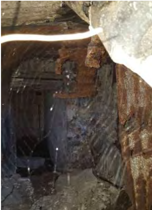
Interior of bunker (seen through gap visible in previous photograph)
