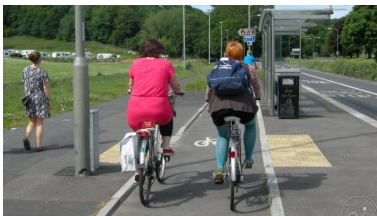
Above: Wide granite kerbs used to define edges of pedestrian realm and the carriageway and withstand level of intensity of pedestrian or heavy vehicle movements and resist damage and misuse. Brighton Station bus interchange, Brighton.
