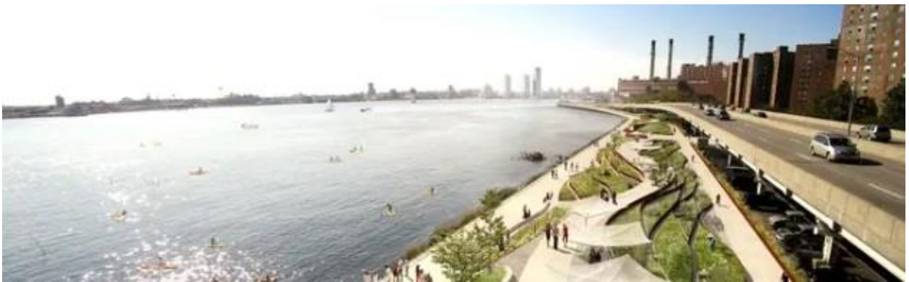
Below: New York's Big U project. Coastline open spaces designed to accommodate floodwater during storms and/or as a result of sea level rise.
