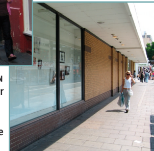
D - DULL Larger units with few doors (2-5 units per 100 m) Little diversity of functions Many closed units Predominantly unattractive facades Few or no details
