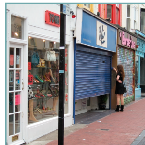
METAL SHUTTERS Unfortunately some of the positive aspects by day are negated at night
