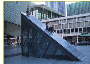
Ground condition of parking garage Schouwburg Plein, Rotterdam, The Netherlands
