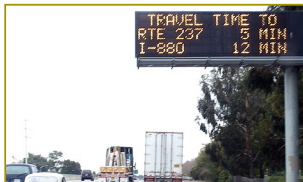
Electronic message signage Highway, USA
