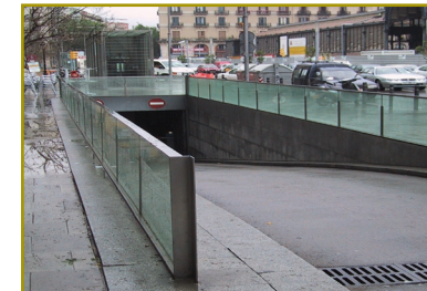
Modern underground garage entrance Barcelona, Spain
