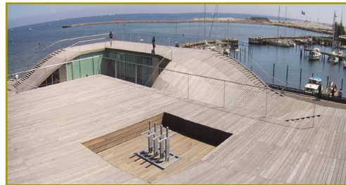
Maritime youth centre linking sea and facilities Copenhagen, Denmark
