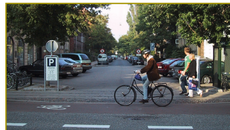
Raised pedestrian crossing Copenhagen, Denmark
