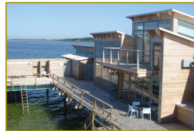
Cafe and sauna facility Bjarred, Sweden
