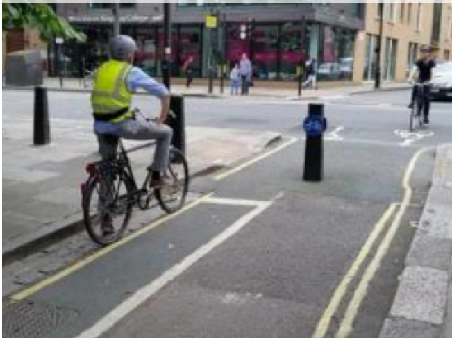
Figure 10.25: Separate cycle phase, Camden
