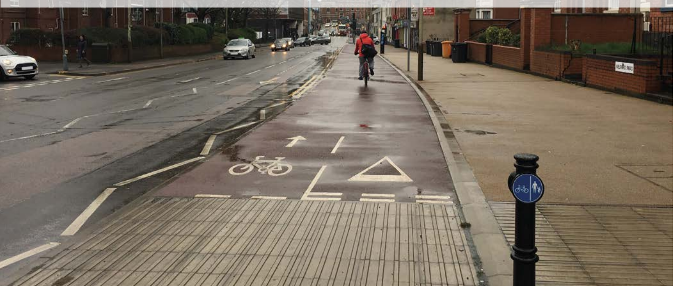
Figure 9.8: Correct use of tactile paving and low kerbs at start of segregated area, Leicester
