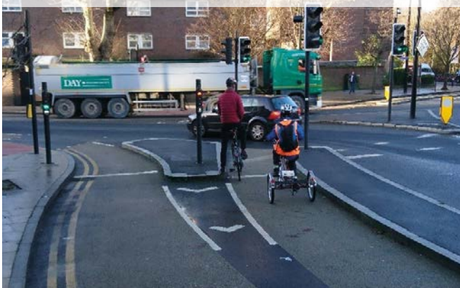
Figure 10.40: Queens Circus roundabout, Battersea
