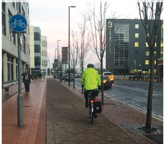
Figure 6.14: Cycle track with sign to TSRGD diagram 955
