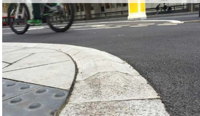
Figure 6.8: Detail of trapezoidal strip and different surface materials for footway and cycle track
