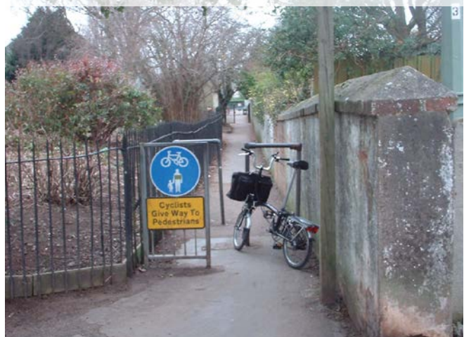
Figure 1.8: Barriers to cycling along a shared-use route (note yellow sign is not permitted in TSRGD)
