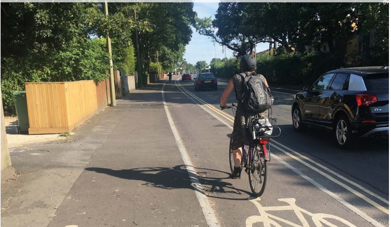
Figure 4.3: Edge of city distributor road, Oxford uses a stepped cycle track for separation from motor traffic
