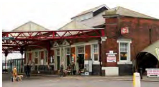
Above - Figure 3.7: Hove Railway Station and footbridge
