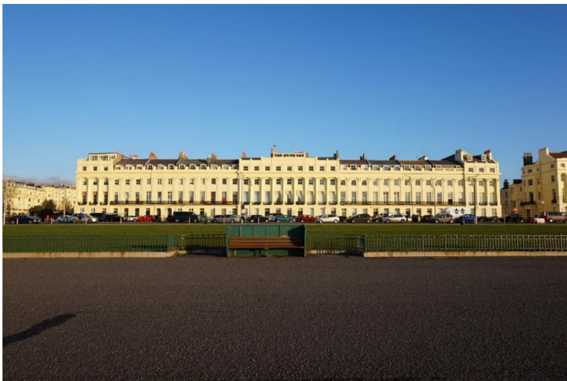
Figure 12: Brunswick Terrace viewed from the southern side of Hove Lawns
