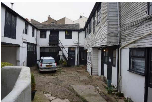
e) Weatherboarded mews buildings, Farm Mews
