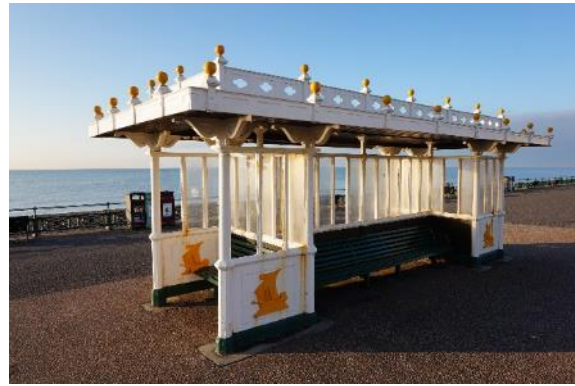
b) Grade II listed shelter
