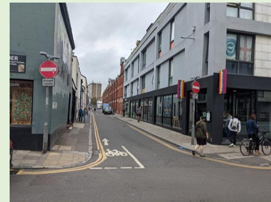
Contraflow cycle lanes (North Laine, Brighton)
