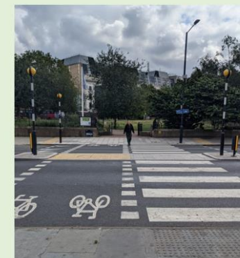
Parallel crossing - Parallel zebra and cycle crossing (Lambeth, London)
