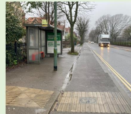
Bus stop boarder, stepped track cycle lane and removal of centre lines (Old Shoreham Road, Hove)
