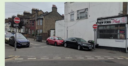
Continuous pavement at side road (Waltham Forest, London)
