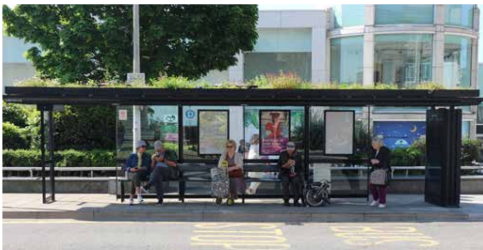
Figure 2.14 shows the newly installed superhub shelter at Churchill Square stop D
