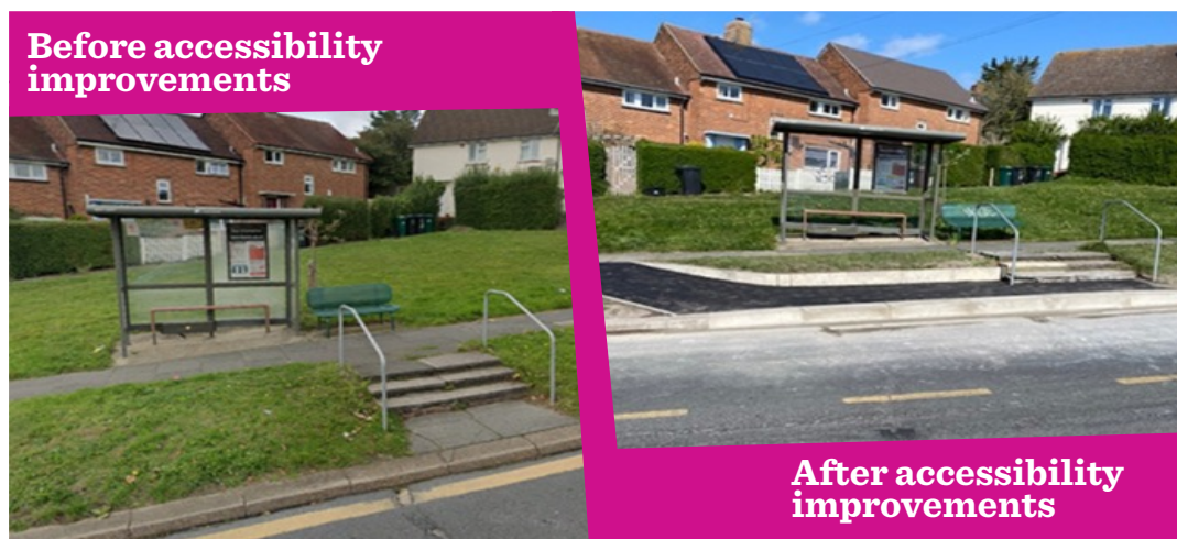
Figure 2.13 shows the northbound Waverley Crescent bus stop on Davey Drive
