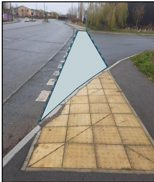
Dropped kerb at junction crossing point with tactile paving
