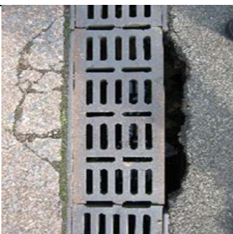
Footway Gap side of Drainage Channel
