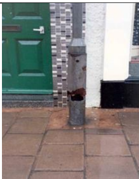
Corroded Column
