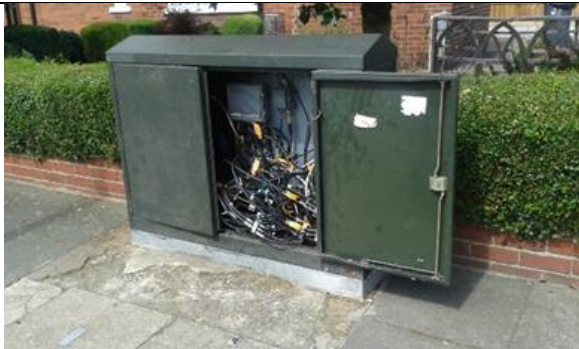
Exposed Wiring
