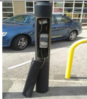
Exposed Wiring
