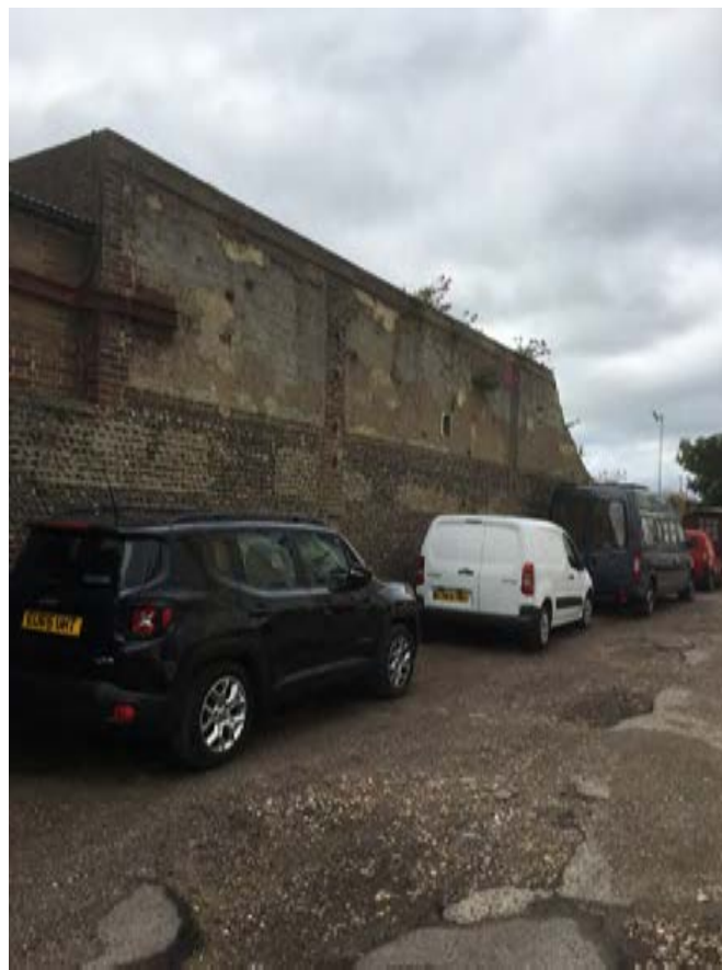
Plate 8: View of part of the western boundary wall
