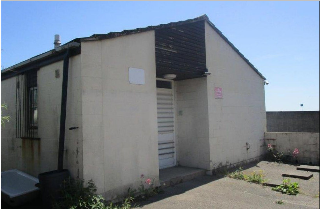
PHOTOGRAPH 5: Exterior of Building B5
