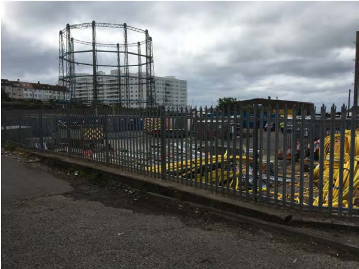
Plate 1: View south across the study site from the northwestern boundary
