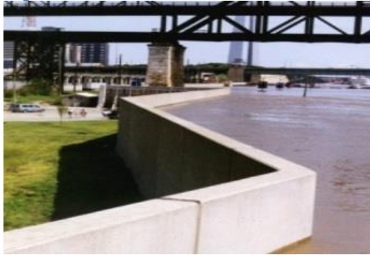
Figure 7.9: Concrete revetment 74
