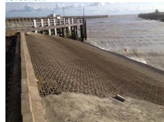
Figure 7.19: Existing defences - concrete revetment 87
