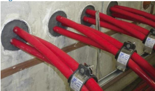
Figure 3.7: Cable duct seal 41
