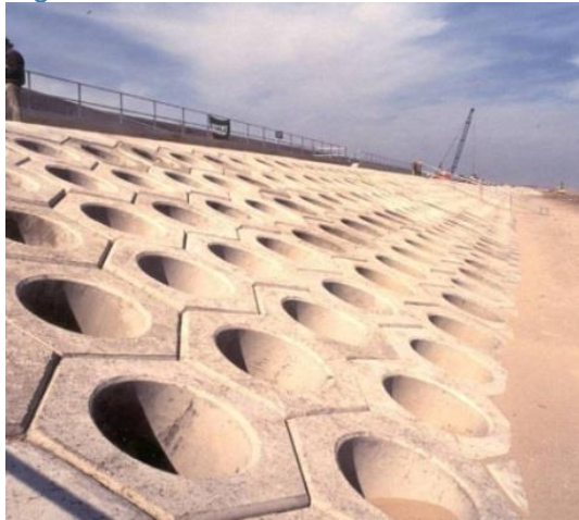
Figure 7.9: Concrete revetment 74
