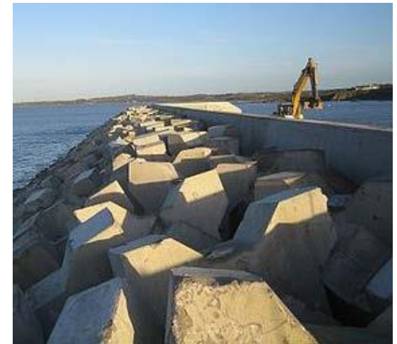
Figure 7.23: Rock revetment with concrete flood wall 91
