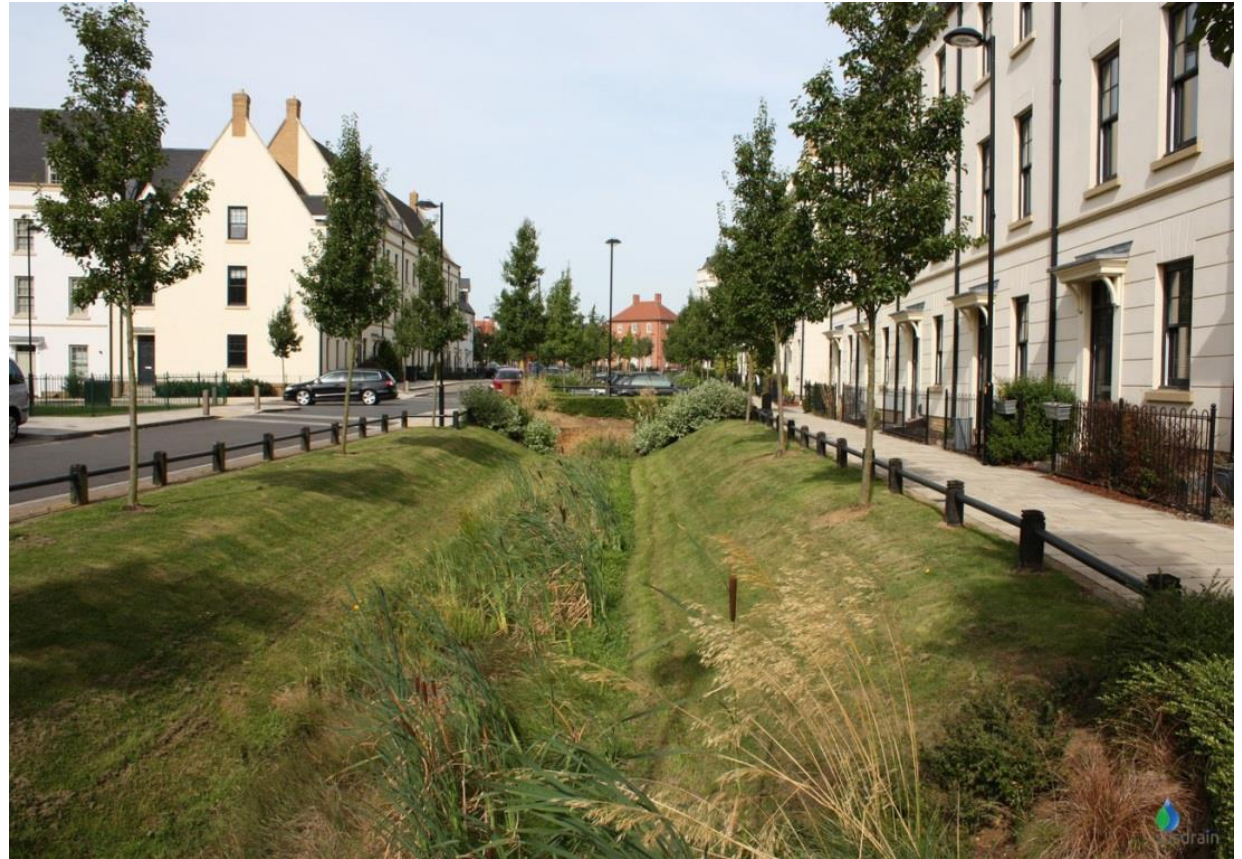
Figure 3.8: Swales at Upton, Northamptonshire 48
