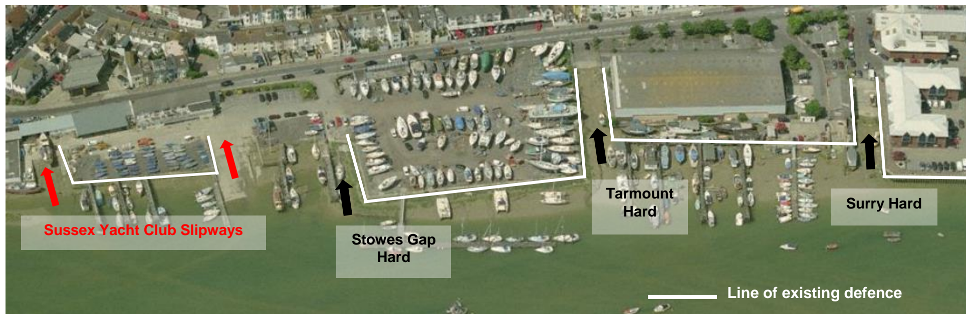
Figure 7.4: Adur Ferry Bridge to Riverside Business Centre - existing defences
