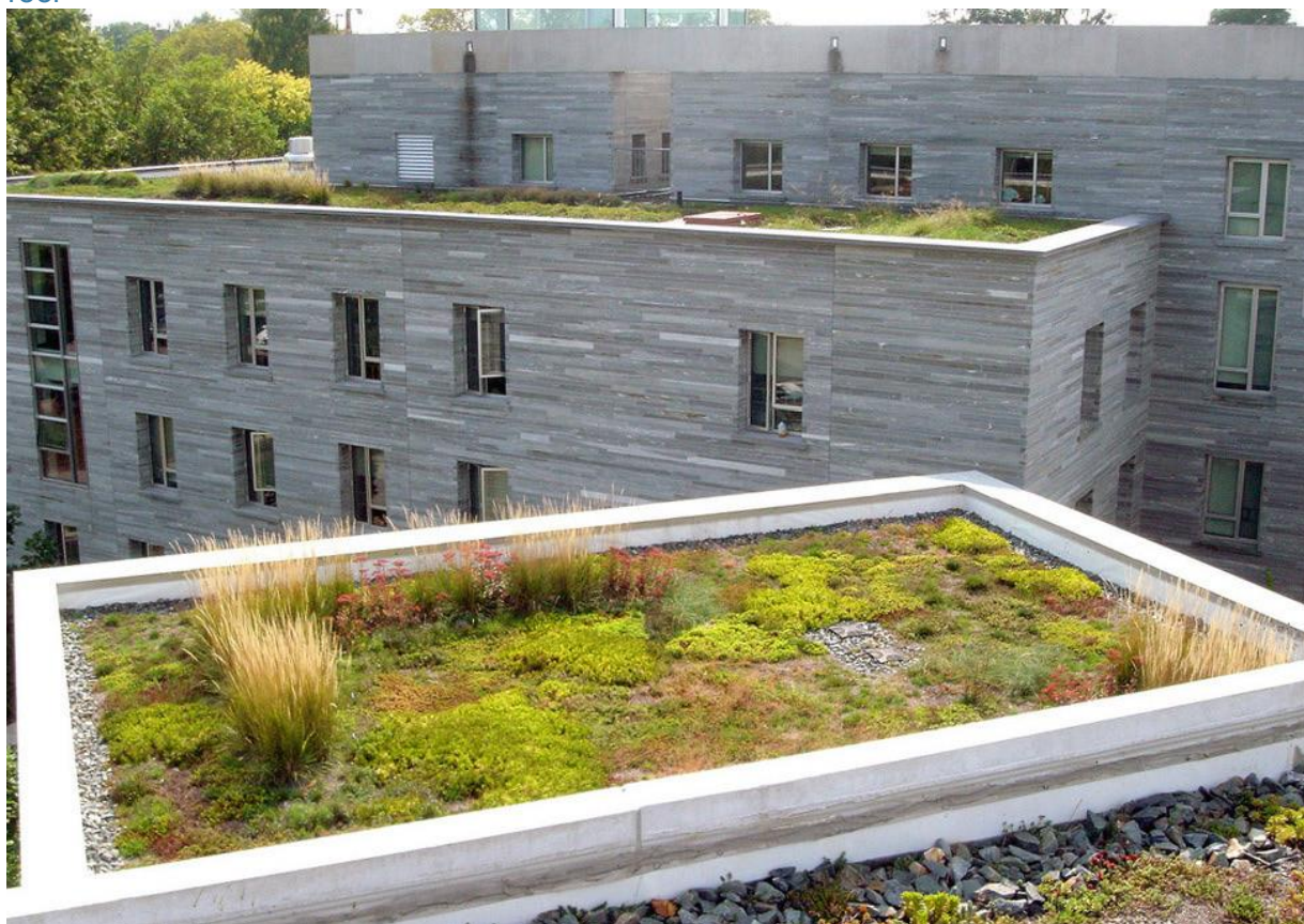
Figure 3.9: Wildflower and sedum green roof 49
