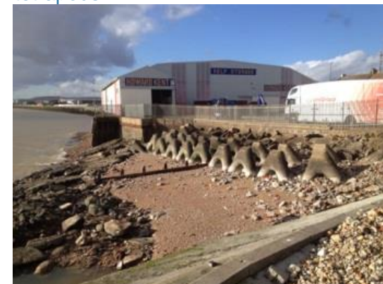
Figure 7.19: Existing defences - concrete revetment 87
