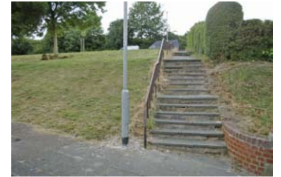
Typical stepped footway linking converging streets
