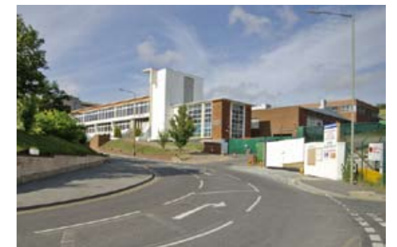
Hollingbury Industrial character area
