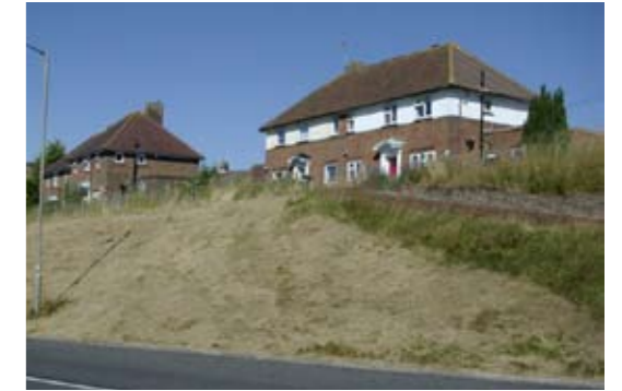
Housing and footway separated from carriageway
