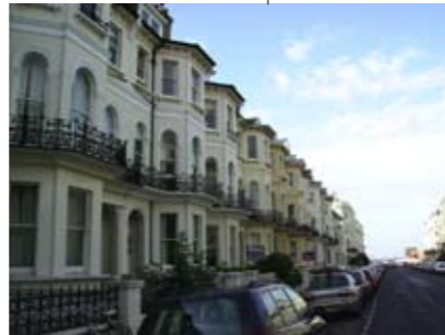
Four storey terraced houses divided into flats: net density = 160 dph
