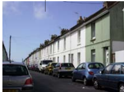
Two storey terraced houses, with small rear patio gardens: net density = 203 dph
