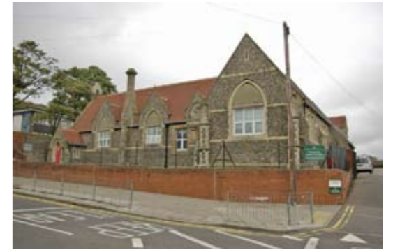
Flint school building, Portslade Village gateway
