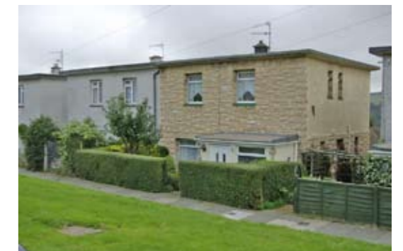
1960s flat-roofed housing
