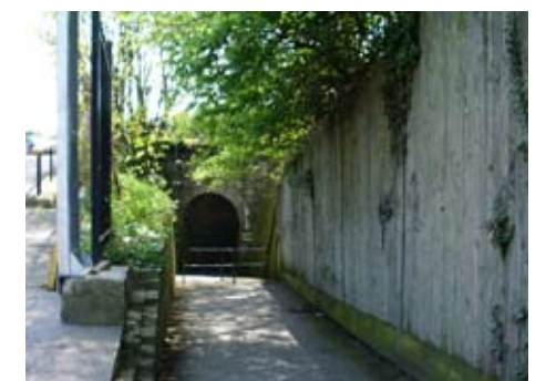
Pedestrian link under railway
