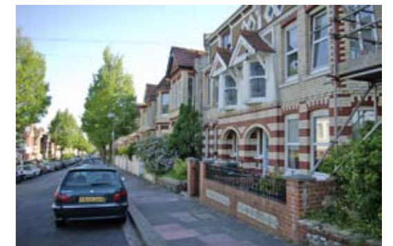
Pre-WWI building facade decoration
