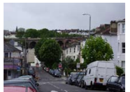
Viaduct character area
