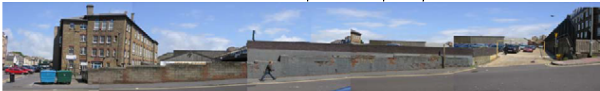
Southern Elevation – Kingswood Street, North
