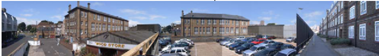
Eastern Elevation – View over site from lane in front of Milner Flats
