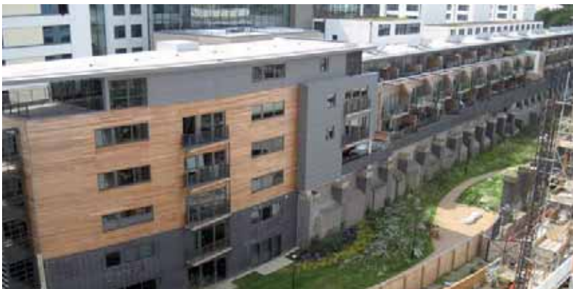
Above: Gladstone Row, Brighton. Thirty one town houses and commercial offices.
