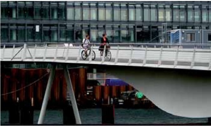
Above: Cycle and foot bridge, Copenhagen, Denmark
